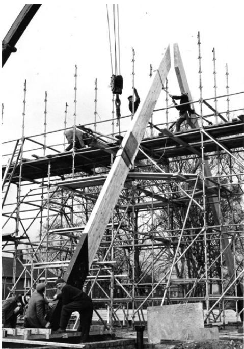
Erecting the beams for the sanctuary area
